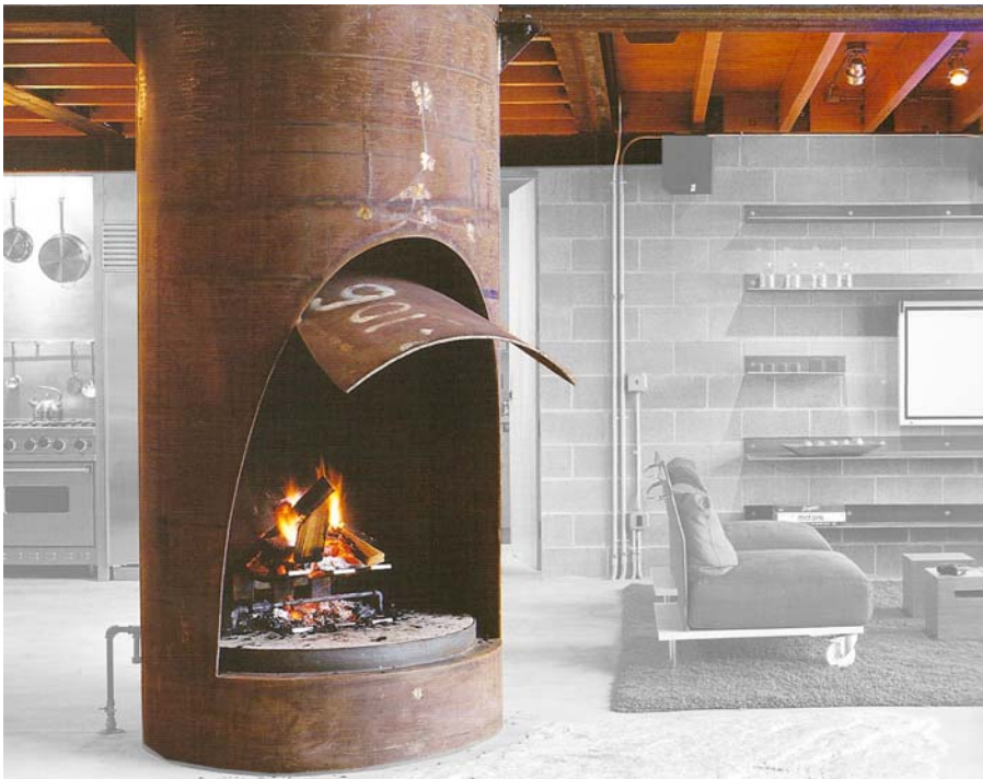
Figure B-6. Structural Fireplace Element. The fireplace serves as a focal point, but also as the central structural post.
