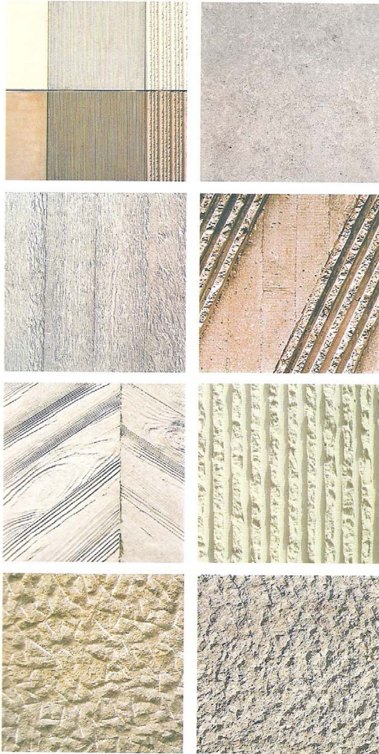
Figure 2-3. Concrete Aggregates, Colors and Textures. (Kind-Barkauskas)
