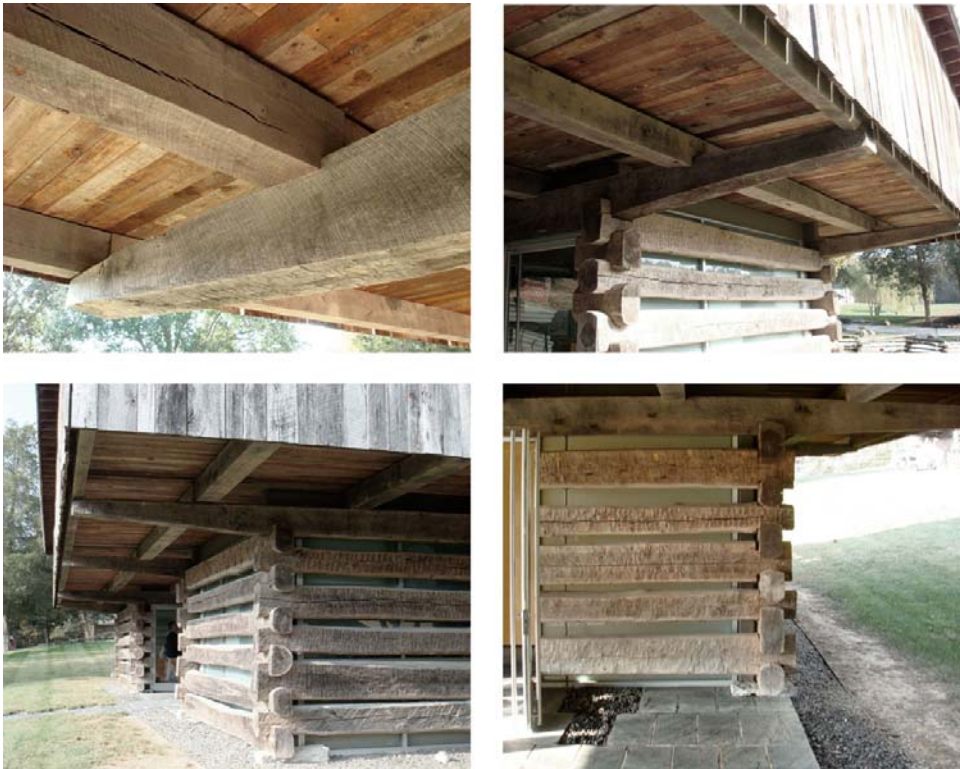
Figure B-14. Cantilevered Barn Details.
