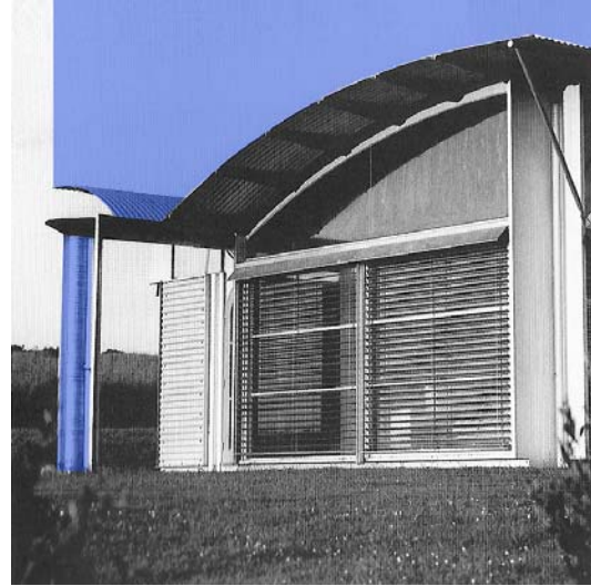
Figure B-10 - The water-collecting roof is a response to the dry climate. The roof collects rainwater and stores it in a cistern. (Phaidon)
