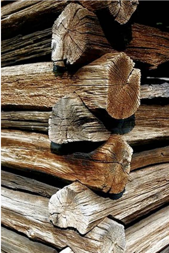
Figure 4-3. Log Joining Detail at Corners. (Dixie)
