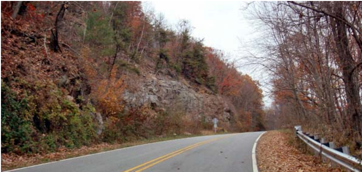
Figure A-4. Town Mountain Road View. (Author)
